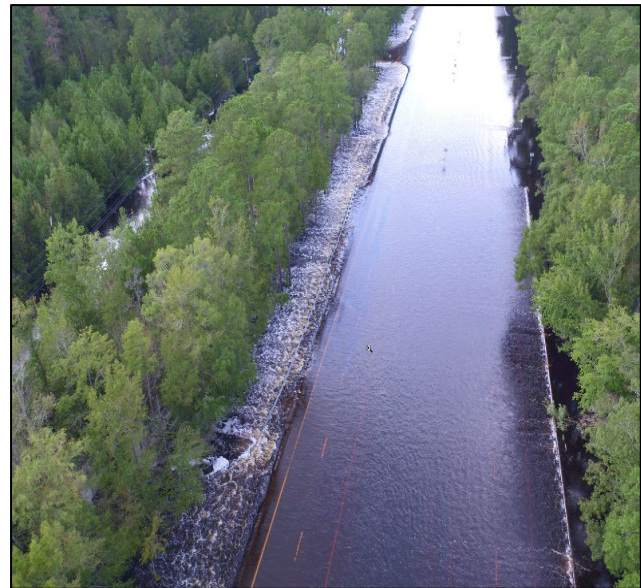
Figure 5: US 74 overtopped from Hurricane Florence, September 2018
