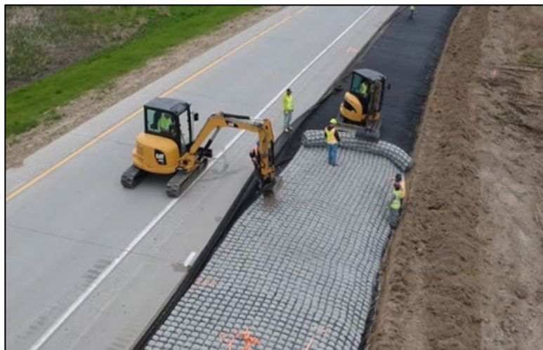
Figure 10: Articulated Concrete Block Mattress (ACBM) installation along shoulder
