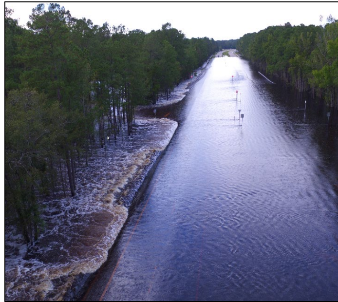
Figure 8: Roadway disruption after Hurricane Florence, September 2018
